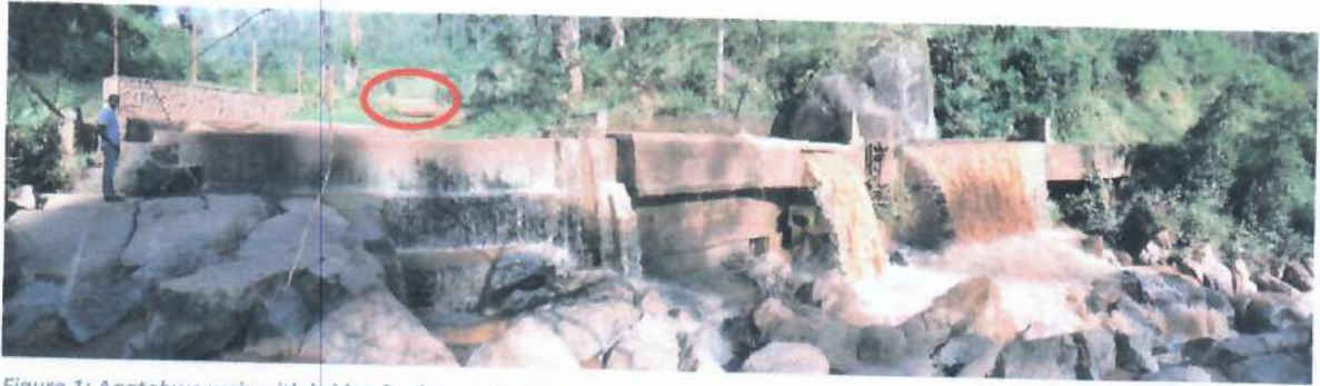
Figure 1: Agatobwe weir with bridge further upstream
