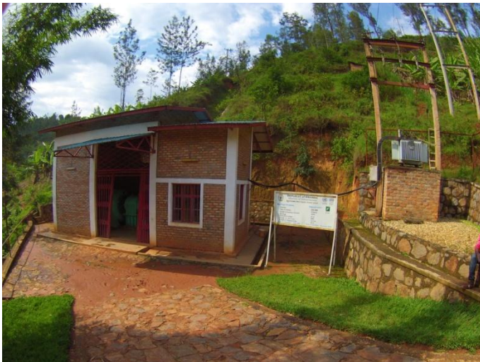
Powerhouse and transformer, south
