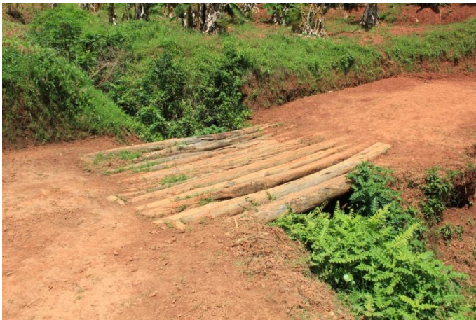
ditch, ph access road
