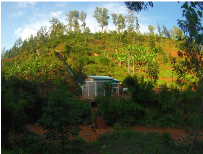
penstock, powerhouse, tailwater
