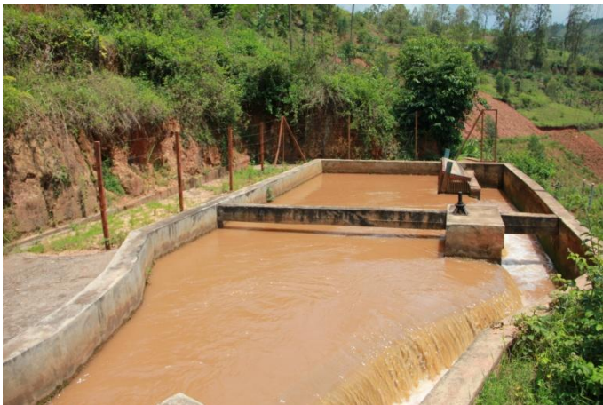
forebay spillway right (4.75 m length)
