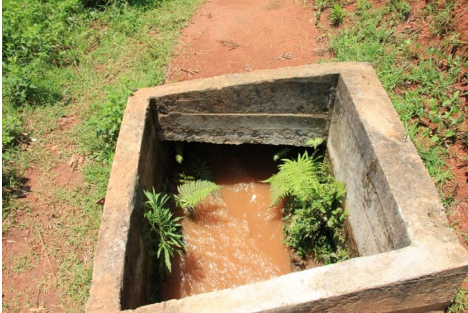
headrace canal, manhole #1, plants, width 1 m, flow depth approx. 0.7 m
