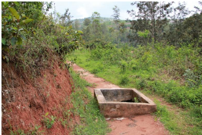
headrace canal alignment, manhole #1
