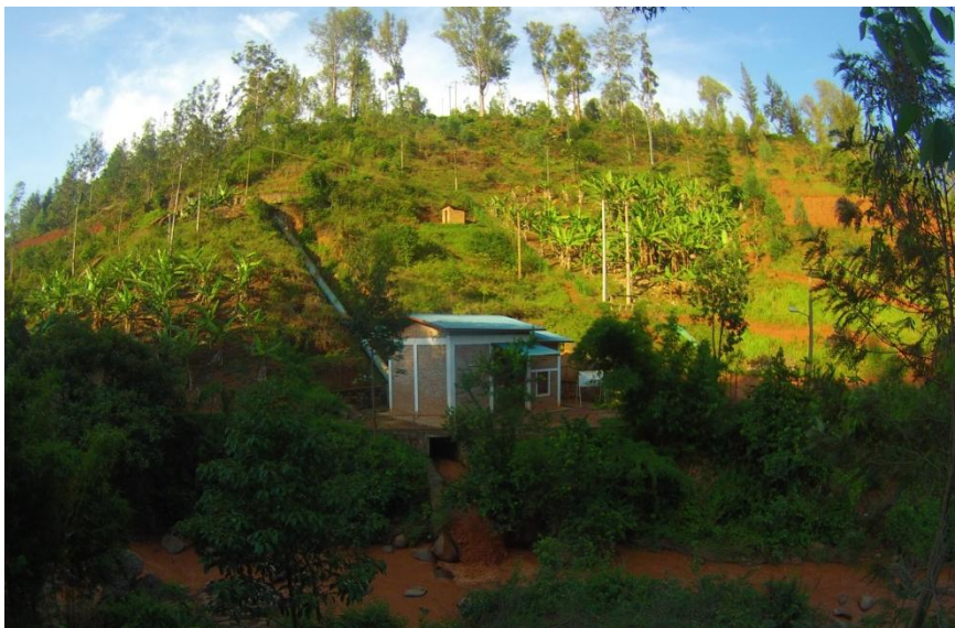
SHPP Agatobwe, RW, penstock and powerhouse
