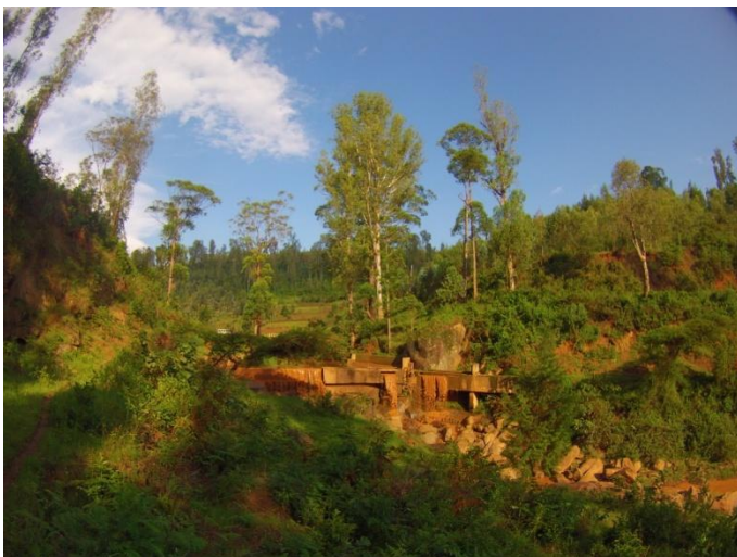
weir, downstream view
