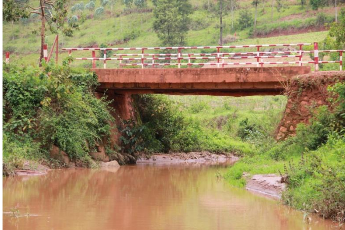
road bridge upstream of weir
