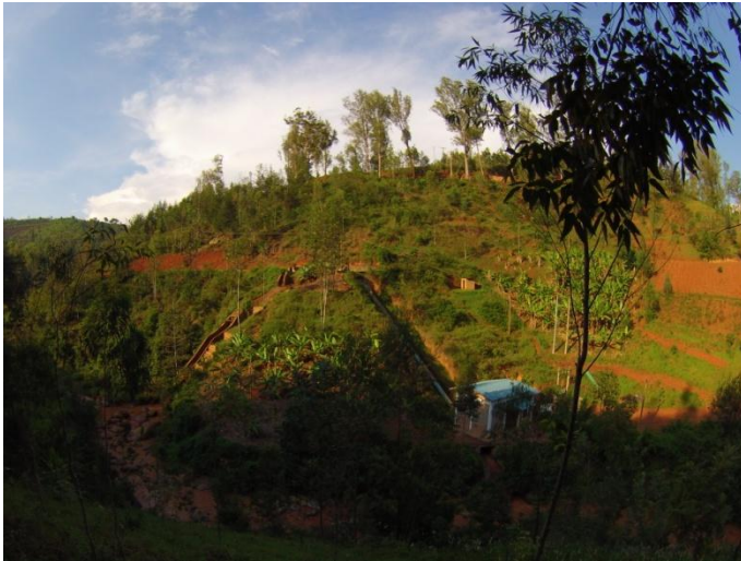
penstock, powerhouse, forebay, spillway
