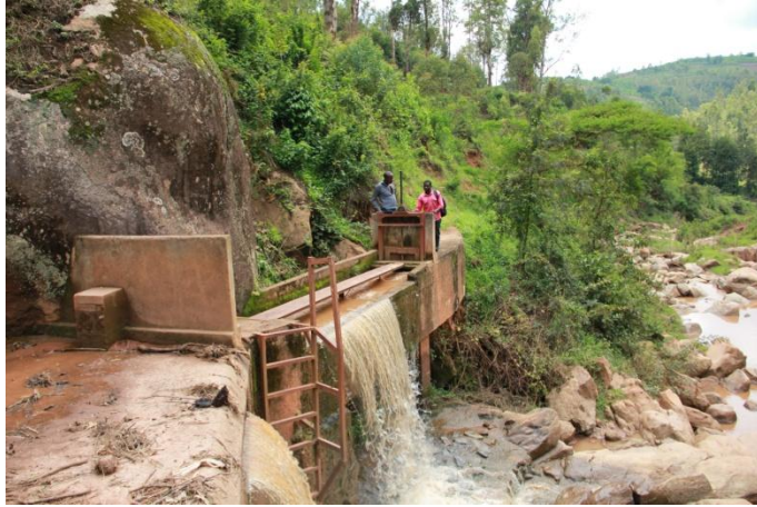
weir, diversion intake, spillway, main gate
