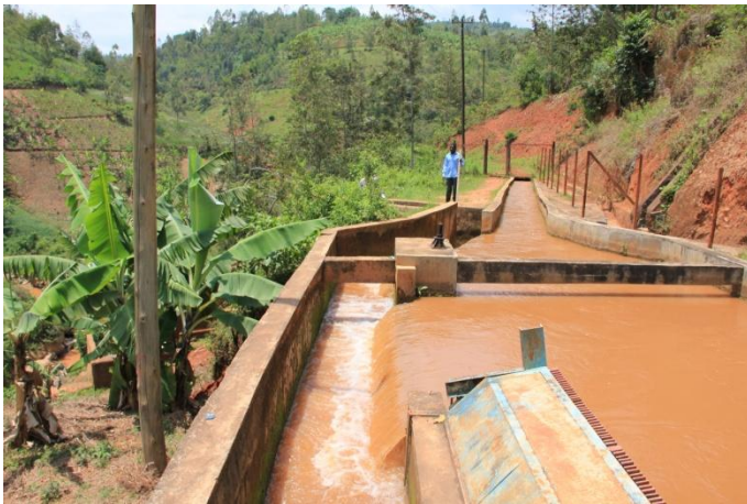
forebay spillway left (3.1 m length)
